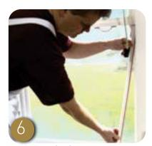
Ease out the bottom two parting beads (C) using a chisel if required.
