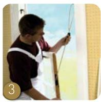
From the Sash Removal System SRS (E), slide out the cord brake (H) from its housing (J) and push up to the pulley. (A)
