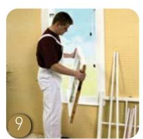
Remove the top sash (F) internally, allowing easy maintenance, cleaning and painting.
