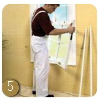
The bottom sash (G) is now fully released and can be easily removed.
