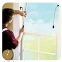
Pull down the top sash (F) and remove the top three pile carriers.
