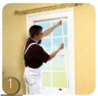
Remove the detachable staff bead(s) (D), unclipping or unscrewing from the middle and working to the top.
